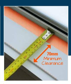
**NOTE**: there needs to be **70mm depth minimum of complete clearance** from any obstacles, from the window frame edge. **Obstacles to look for**: Mullions, Locks, Window Handles, Winders, Storm Bars etc
