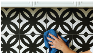
Scrub tiles before applying topcoat
