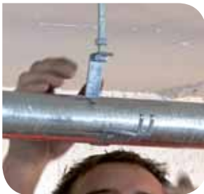
4. Finish off row and simply hang pipe on bracket, SPEED Clip will hold pipe temporarily allowing final adjustment.
