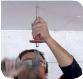
1. Measure off and fit bulldog fastenings.
