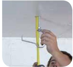
3. Measure fall and spin on top nut approx 5mm above the measure.
