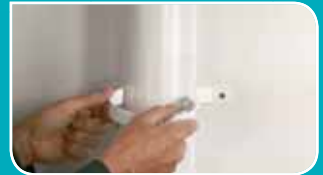
3. Place pipe into bracket base
