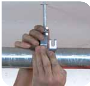
5. Then simply fold SPEED Clip arm upwards and 'snap' into place to lock shut.
