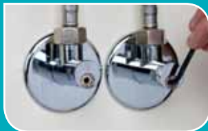
Install Iso-Filter and/or Iso-Adaptor if required.
