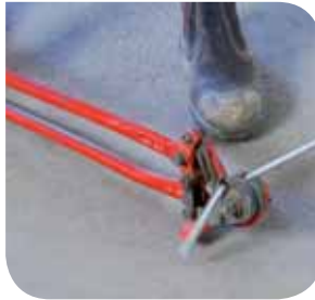
2. Trim All Thread and secure to masonry anchor point.
