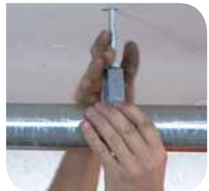
6. Tighten top nut to secure.
