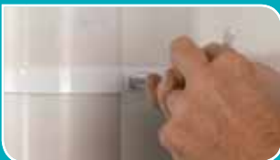
4. Secure front of the brace with bolt & nuts (supplied)
