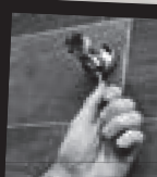
Wind on wall bracket using a screwdriver
