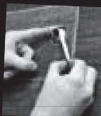
Apply teflon tape anti-clockwise onto wall outlet
