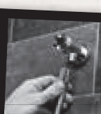
Push back wall cover flange and attach hose
