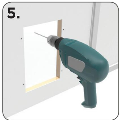
5. Check outer frame fits opening and screw holes align. Drill each of the screw holes using a 8mm bit.
