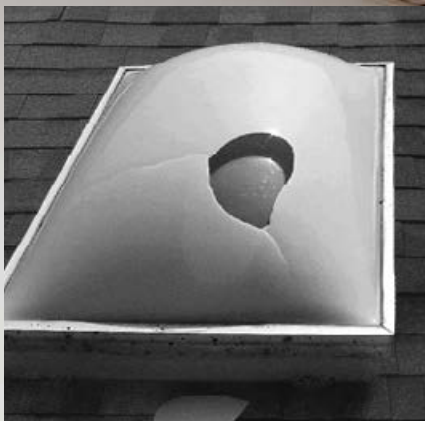
Old acrylic domes can be easily damaged
