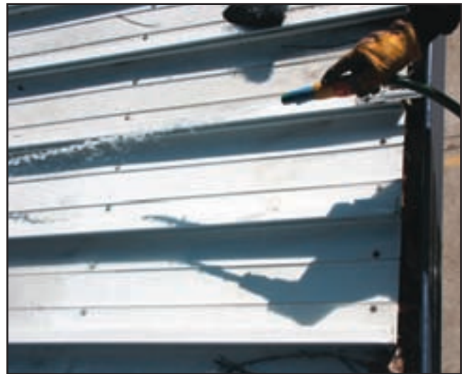
2) Use a hose to blow away twigs and soften hardened dirt.
