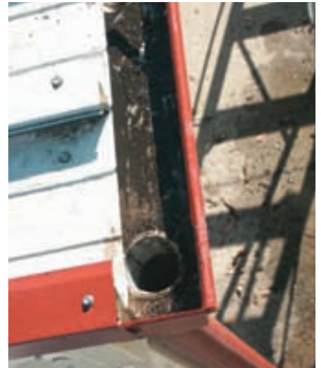
3) When litter is removed, the layer of hardened dirt is revealed below.
