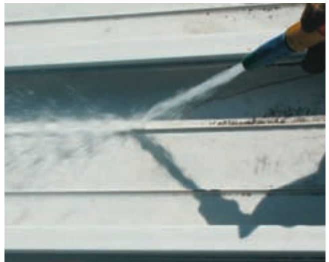
4) The roof cladding should be clean after you rinse.
