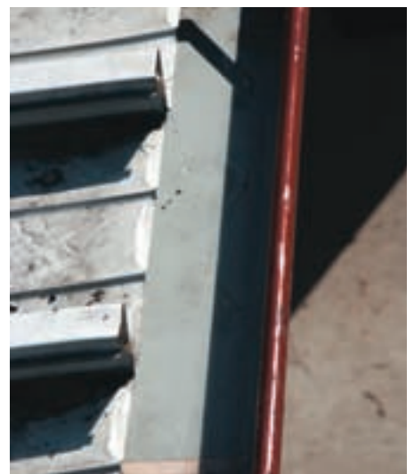
6) When the gutter has been cleaned, it should look like this.
