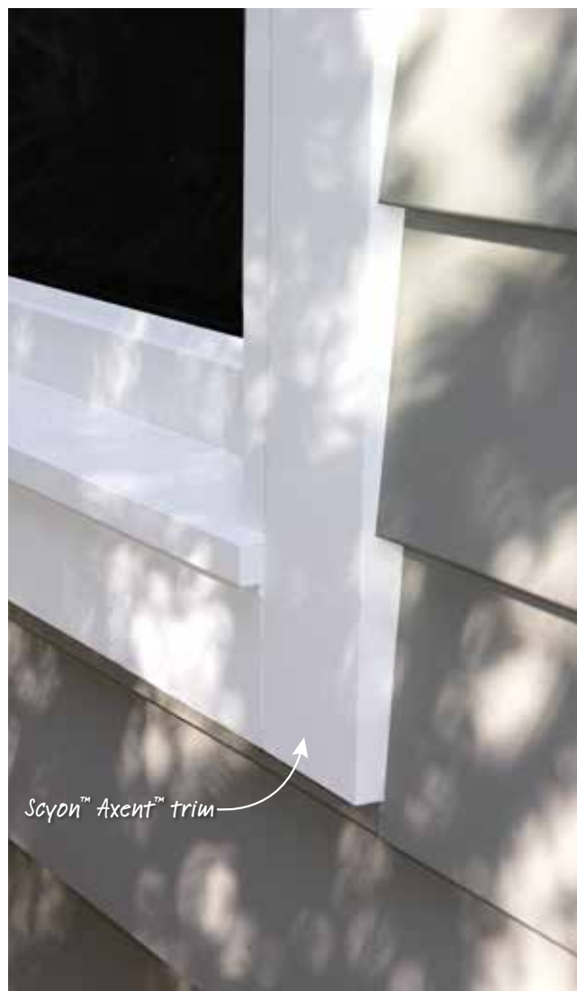
38mm Scyon™ Axent™ trim fixing around window
