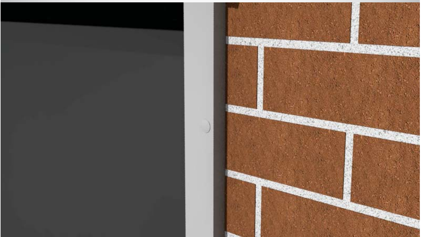
24. After putting all the screws in, use the plastic caps to cover the holes.
