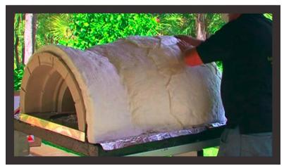
Start at the front, finish at the back ensuring complete coverage. Excess insulation must be used to plug gaps. Cut a hole for the flue.
