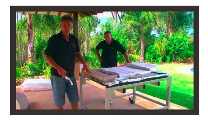
Install ovens floor insulation blanket and flatten down tightly.
