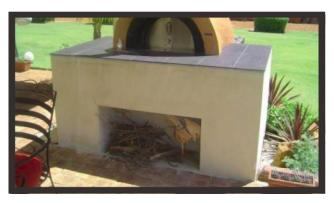
The concrete slab (top of base) must be dry, level and clean before commencing oven construction. A concrete sealant is recommended to prevent the oven drawing moisture from the base.
