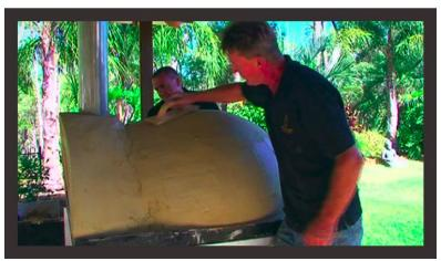
**Insert the flue into the front chamber hole with the seam of the flue facing the back of the oven before beginning the rendering process**. Use a spirit level to ensure the flue remains straight. For best results, use a steel float to apply the render mix. What can go wrong?
