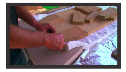
Measure back from front floor piece 655mm. Mark foils both sides of slab.
