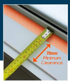
**NOTE**: there needs to be **70mm depth minimum of complete clearance** from any obstacles, from the window frame edge. **Obstacles to look for**: Mullions, Locks, Window Handles, Winders, Storm Bars etc
