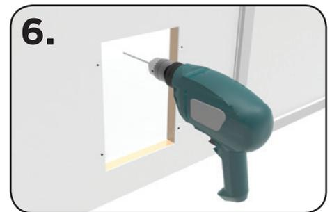
6. Check outer frame fits opening and screw holes align. Drill 3mm pilot holes.
