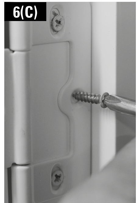
Hinge locking screw
