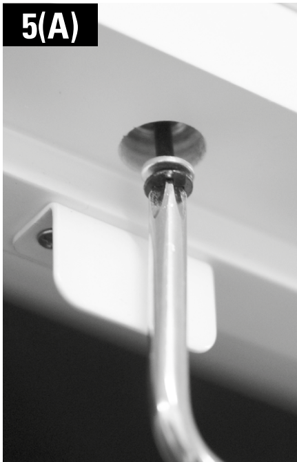
Secure frame with remaining screws
