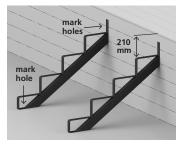
Determine the location of all stringers and ensure the top tread support is 210 mm down from upper deck surface. Then, for each stringer, level and mark the two fastener locations on the deck rim, and one fastener location on the lower deck surface.
