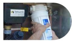
ACTION: Turn off the power point, close mains water valve, unscrew body of cartridge filter, remove cartridge filter and replace it, ensure the cap is tightened.
