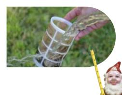
Action: turn off pump power, unscrew filter body, remove filter and clean & replace.
