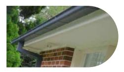
The gutters on house capture the rainwater running off your roof. These gutters direct the rainwater to the downpipes which in turn feed into the rainwater collection tank. It is important that these gutters are kept clean and in good order.
