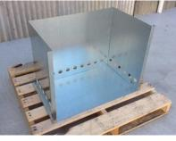
Step 4: Screw 8"collar in place.30mm edge to front for 200i.83mm edge to front for 300i.
