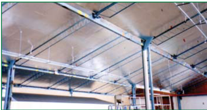
KOOKABURRA MANUFACTURING PLANT- REFURBISHMENT Here FOILBOARD® INSULATION PANEL was used to drastically improve the thermal efficiency of this factory. The pure aluminium foil laminated to FOILBOARD® also helped increase the ambient light whilst adding to the aesthetics.
