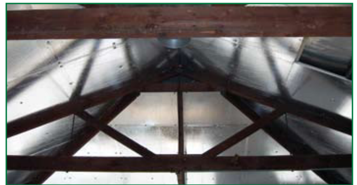
B.P.S. Technical Bookshop FOILBOARD® INSULATION PANEL was used here to retro fit an old storehouse to a retail outlet. The developers were keen to maintain the industrial look of the building whilst drastically improving thermal efficiency.
