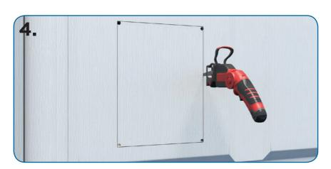
4. Using a reciprocating jigsaw, cut out the opening, cutting along the pencil outline. Check frame fits opening.
