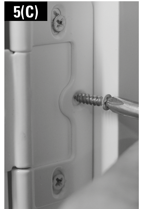
Hinge locking screw
