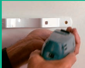
Step 2 – Position bracket and fasten to wall.
