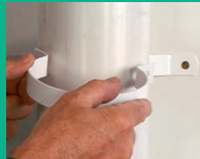
Step 3 – Place pipe into bracket base.
