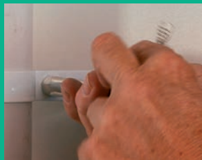
Step 4 – Secure front of the clips with bolt and nuts (supplied).
