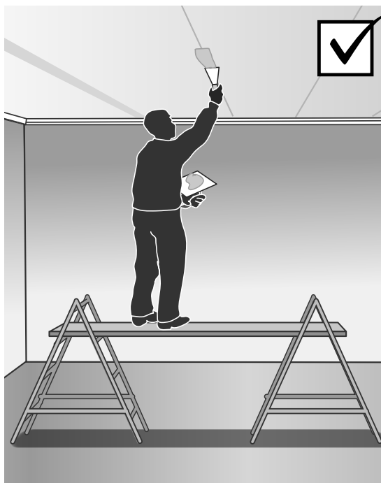
Figure 26 (b) A safer alternative: plasterers' trestles
