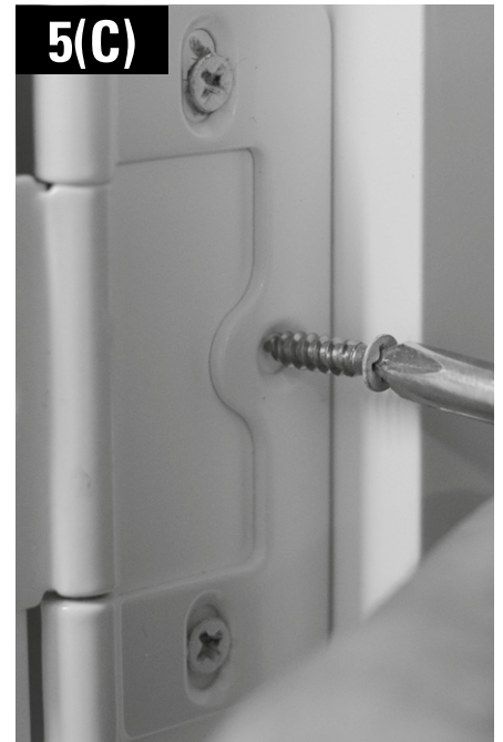
Hinge locking screw
