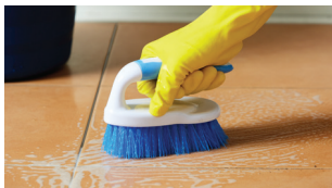
Scrub tiles before applying topcoat
