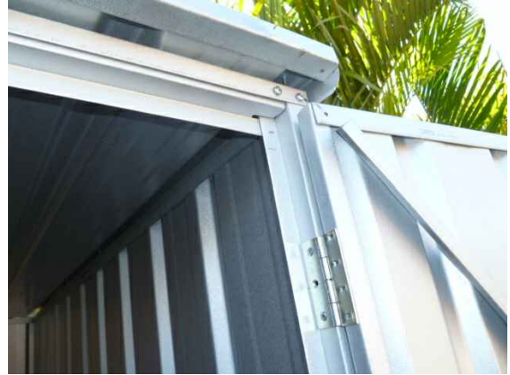
DOOR CONNECTION & JAMB ASSEMBLY
