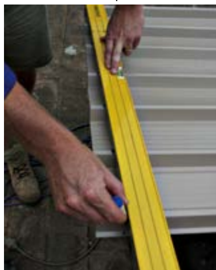
Measure the amount to be cut and mark the sheet. Ensure you measure edge to edge, not rib to rib.
