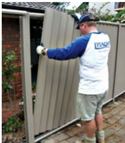
Position 3rd sheet. Gentle force can be used.
