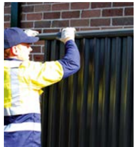
Lift top rail and rotate until all infill sheets slide into rail. Tap top rail down but do not fasten into position yet.
