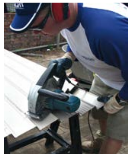
Cut the infill sheets three at a time. This equals a single bay and ensures uniformity. Measure twice, cut once.
