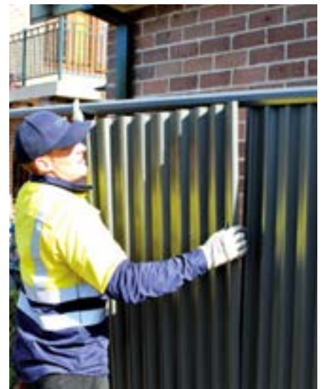
Place 2nd & 3rd sheets into bottom rail, ensuring there is sufficient overlap.
