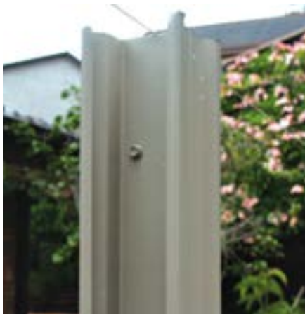
Use stringline to set post heights.
