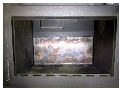
Hot water generator in position
