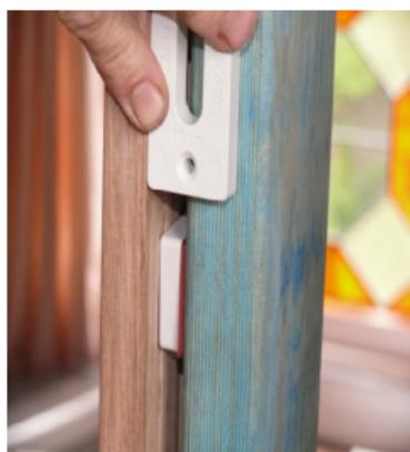
Now reposition jamb and check the front edge of the jamb is set 10mm proud of the wall frame to allow for standard 10mm plasterboard cladding. If different cladding
