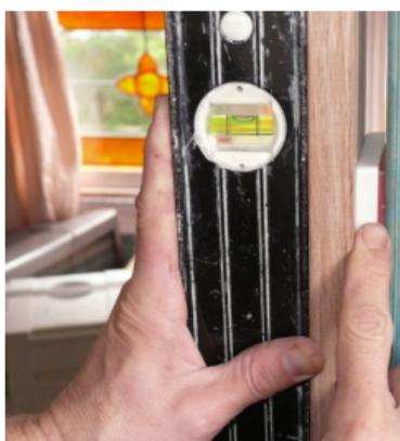
The loose fitting jamb will allow for adjustments to be made for any distortion in the wall frame and to be sure the jamb is plumb. Use a level to check each side and place packers
