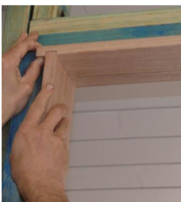
Lift and position the jamb assembly into the wall frame. (Note: this will be a loose fit and clamps or wedges may be required to hold jamb until it is affixed.)
