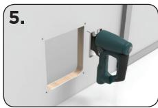
5. Using a reciprocating jigsaw, cut along marked lines.
