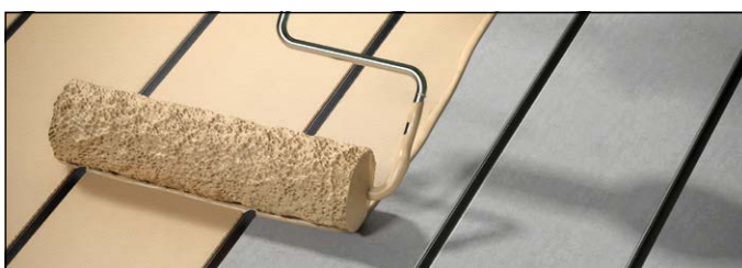
FIGURE 15 APPLY EXTERIOR TRAFFICABLE PAVING PAINT OR SEALER
