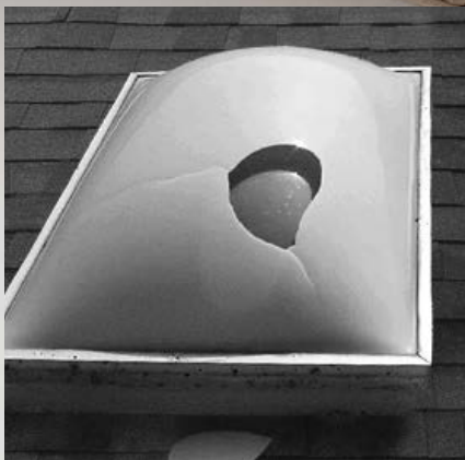
Old acrylic domes can be easily damaged
