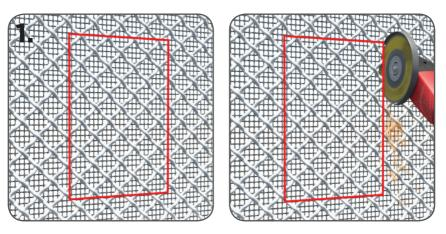
1. Take the measurements needed to cut the opening by following steps 1-3 of the previous instructions. Using an angle grinder, cut out the opening.
