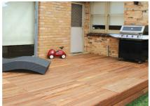
The good times modular deck system can be installed directly onto any existing surface. Simply construct the pre-fabricated frames, fit the supports and adjust heights to match uneven surfaces. Then insert the pre-fabricated merbau deck panels. Use a concrete paver when positioned over soft surfaces.
