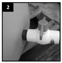
Connect the 25mm Ball Valve to the outlet of your rainwater tank.
