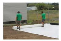
Depending on the soil type and loading, a geotextile is recommended to be laid on the sub-grade surface.
