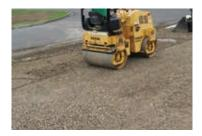
3 Compact a suitable base course material to sufficient depth, ensuring that the area is shaped to prevent ponding.
