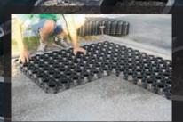
Lay panels ensuring they are interlocked correctly. Trim to shape with a circular saw, or similar, where required. On steep slopes or heavy turning areas use steel anchors.
