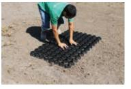
Lay panels ensuring they are interlocked correctly. Trim to shape with a circular saw, or similar, where required.
