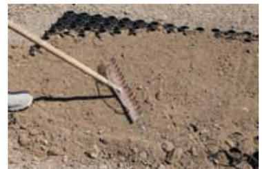
**6** Fill with good screened topsoil up to 10mm above the top of the panels and sow grass or lay instant turf.
