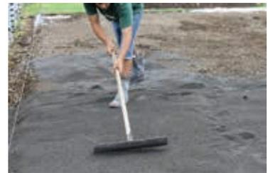
**6** Place a 25mm bedding layer of clean, sharp sand over the base course layer and screed to level.
