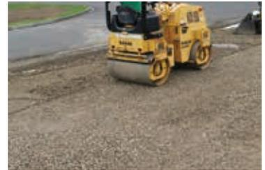
**3** Compact a suitable base course material to sufficient depth, ensuring that the area is shaped to prevent ponding.
