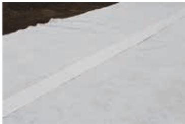
**4** A geotextile can be laid on top of the base course as a separation layer between the base course and sandy top soil bedding layer to prevent migration of the particles.\*
