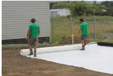
**2** Depending on the soil type and loading, a geotextile is recommended to be laid on the subgrade surface.\*
