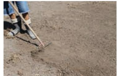
**4** Use good screened topsoil or sand and spread a thin layer over prepared base to create an even bed.
