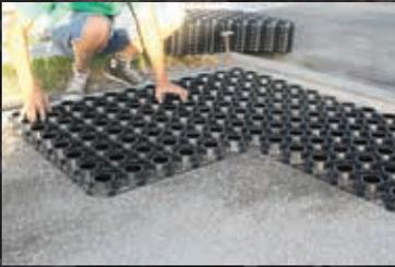
**7** Lay panels ensuring they are interlocked correctly. Trim to shape with a circular saw, or similar, where required. On steep slopes or heavy turning areas use steel anchors.
