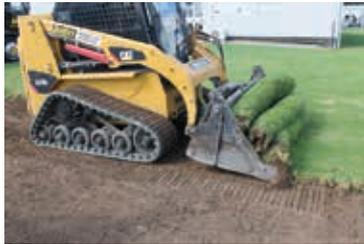
**1** Excavate ground shape and level to achieve sufficient grading and load bearing.
