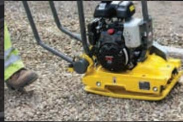
**9** Use a plate compactor to consolidate the filling material into the panels. Fill any voids that show with more aggregate. Filling material should just cover pavers.
