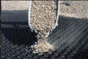
**8** Fill the panels with specified angular roading aggregate or decorative gravel to finished levels (7mm - 19mm aggregate size is recommended).
