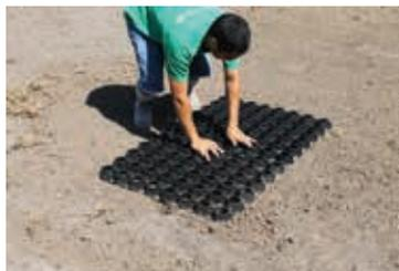
**5** Lay panels ensuring they are interlocked correctly. Trim to shape with a circular saw, or similar, where required.
