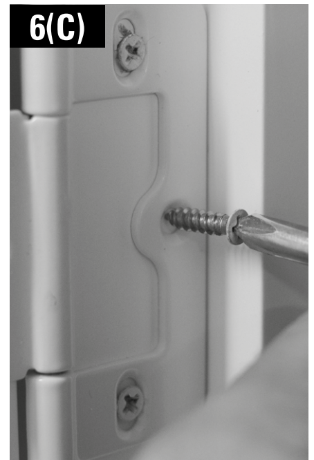
Hinge locking screw
