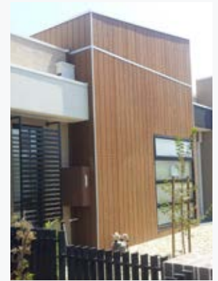
4 MONTHS: The board shows signs of lightening.
