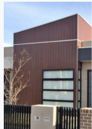
COMPLETE: After 3 coats the timber is restored and is now UV protected.
