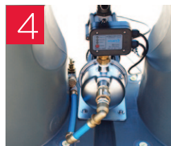
Pump installed with rain/mains changeover
