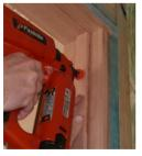
Finally cut and fit the door stop beading using the line drawn earlier as a guide. Hang door and fit door furniture before cladding wall and fitting architrave. The inner edge of the
