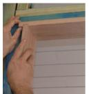
Lift and position the jamb assembly into the wall frame. (Note: this will be a loose fit and clamps or wedges may be required to hold jamb until it is affixed.)
