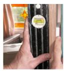
The loose fitting jamb will allow for adjustments to be made for any distortion in the wall frame and to be sure the jamb is plumb. Use a level to check each side and place packers
