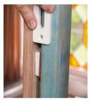
Now reposition jamb and check the front edge of the jamb is set 10mm proud of the wall frame to allow for standard 10mm plasterboard cladding. If different cladding
