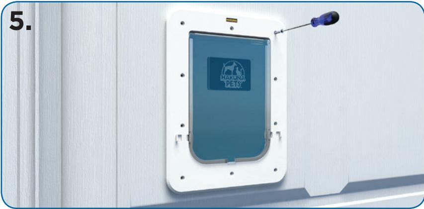
5. Align tunnel (if required) and frames into the opening and secure with screws and caps provided. Select the correct size screws below for your installation.
