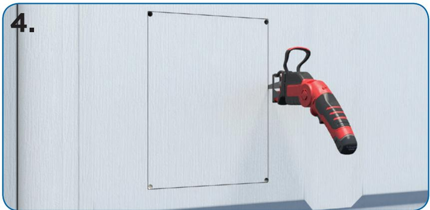
4. Using a reciprocating jigsaw, cut out the opening, cutting along the pencil outline. Check frame fits opening.
